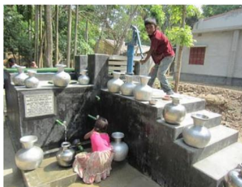
④砒素鉄除去装置(AIRP)
